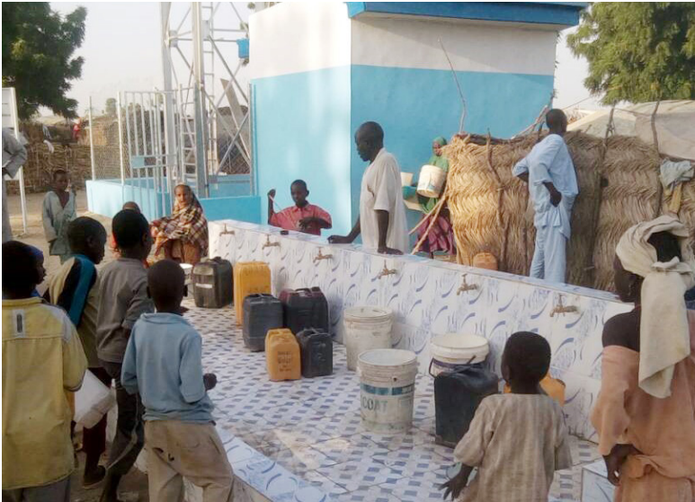
Completed solar-powered borehole at Elbadawi Camp, Muna Garage
