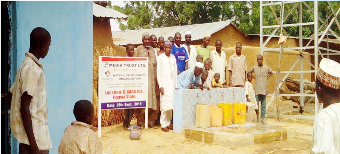
Borehole constructed at Gada LGA, Jigawa State
