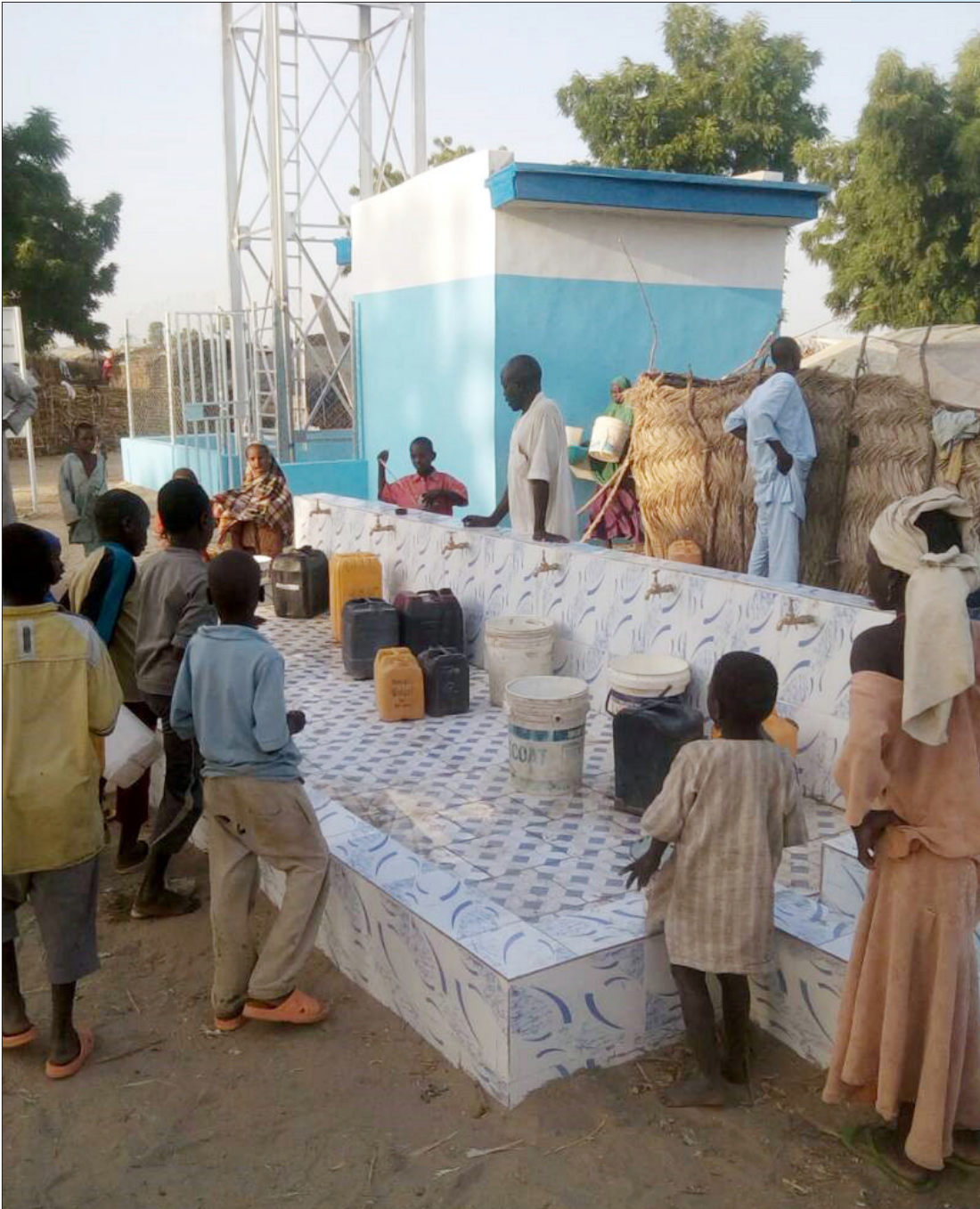
Completed solar-powered borehole at Elbadawi Camp, Muna Garage, Maiduguri, Borno State
